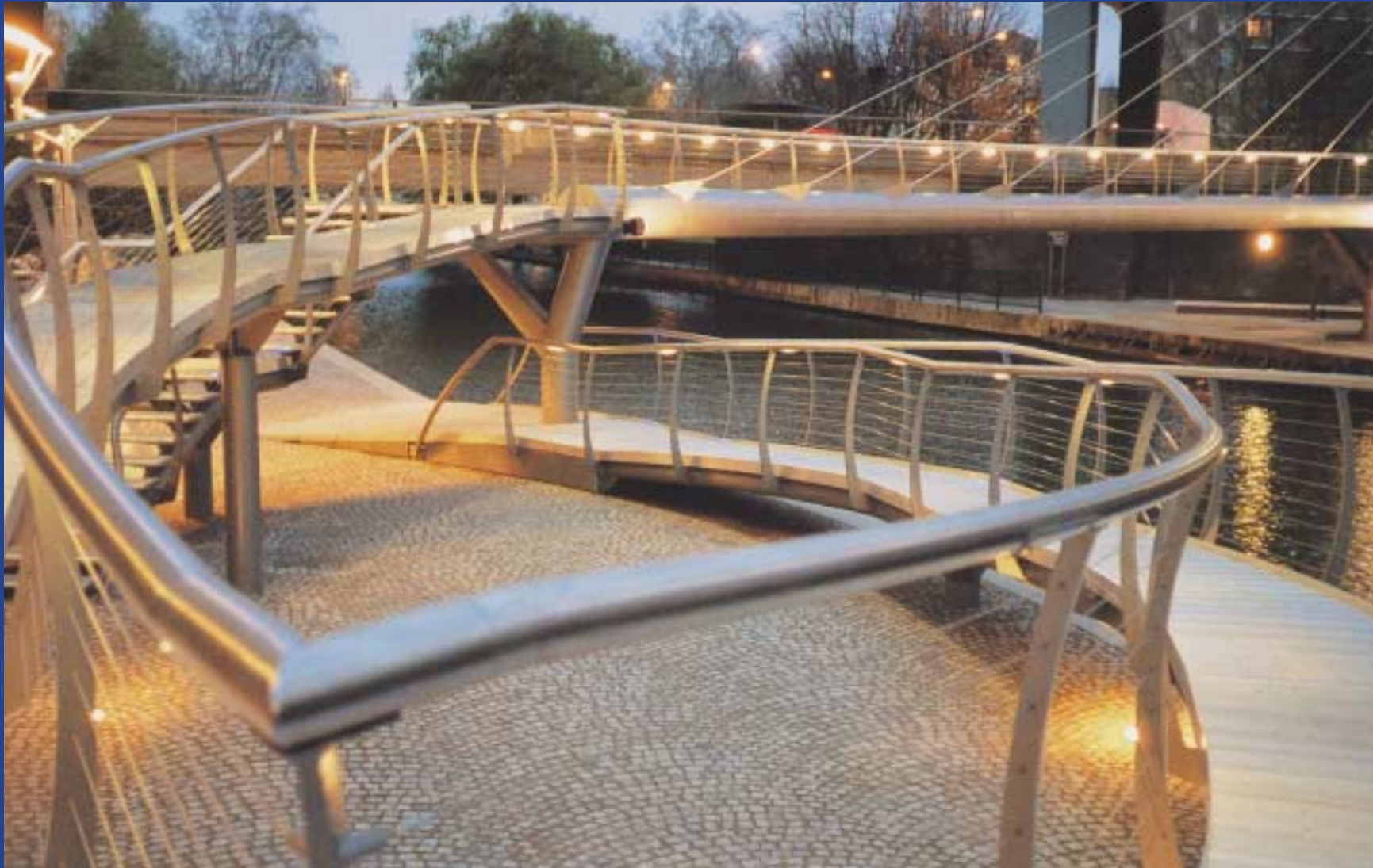
Footbridge at Paddington Central The Paddington Central footbridge enhances the permeability of the site, allowing the public access to the canal towpath at Paddington for the first time ever.
